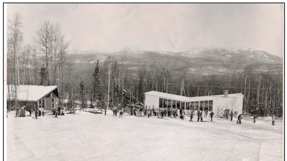
First wing of the second base lodge - c. 1960
